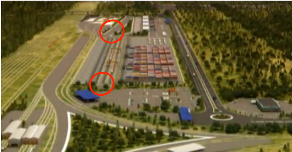
Photograph 1: Hasanbey Centre lacking connection
